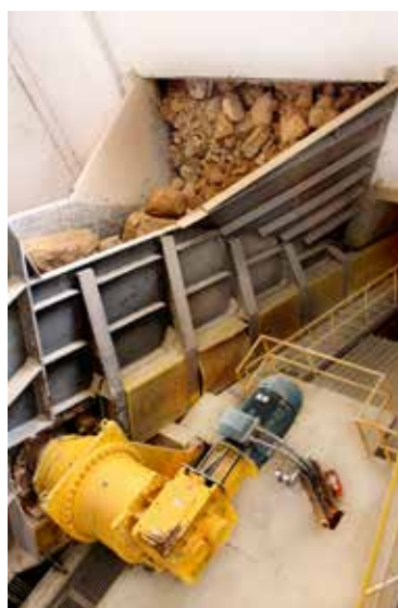
Bulk cement unloading from vessel packing plant
