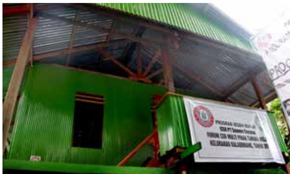
Bedah rumah penduduk miskin Houses renovation for the poor
