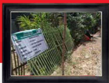
Agustus August Pembuatan Drainase. Drainage construction.
