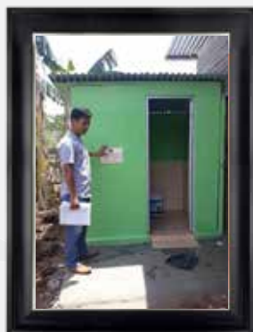
September MCK bagi masyarakat. Latrines Construction.
