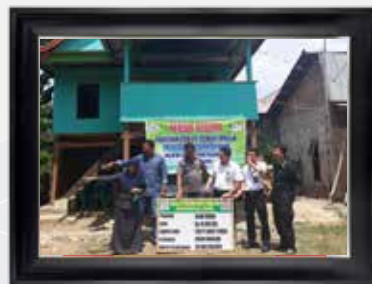
September Bedah Rumah 2. House Renovation 2.
