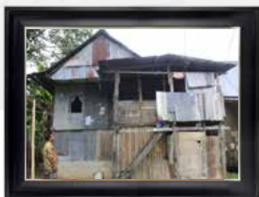
September Bedah Rumah. House Renovation.
